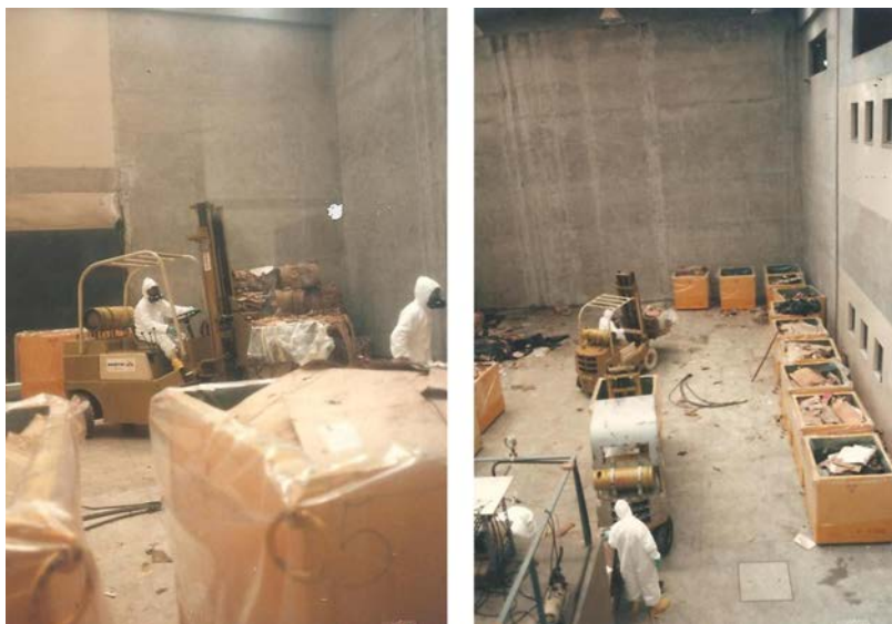
Figure 2 - Contaminated paper bales collected and stored in the waste boxes in August 1988.
